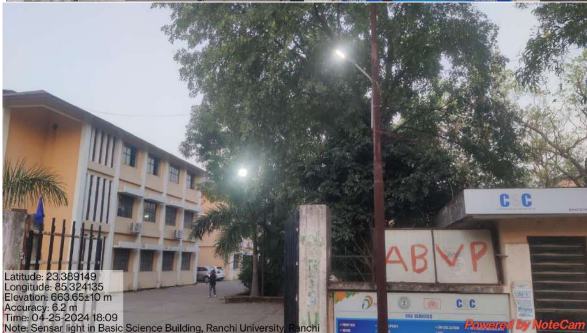
Fig. Sensor Light installed in the campus of Ranchi University, Ranchi (Basic and Applied Science Building, Ranchi University, Ranchi).
